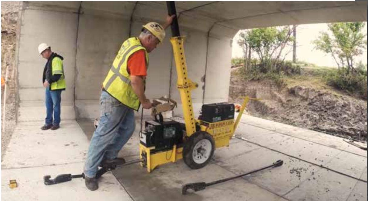
This picture shows the procedure for locking the puller into place prior to pulling.
